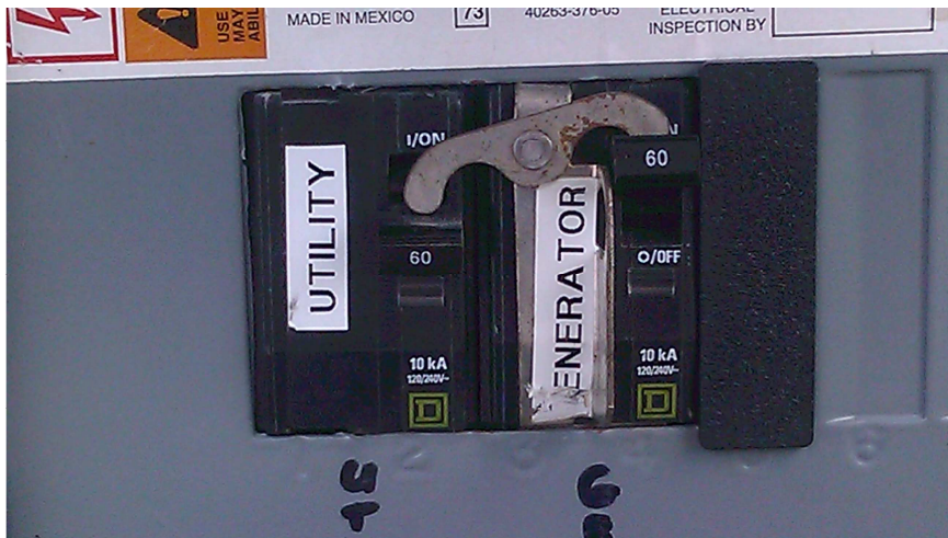
Figure 10. Breakers on Generator Power.
