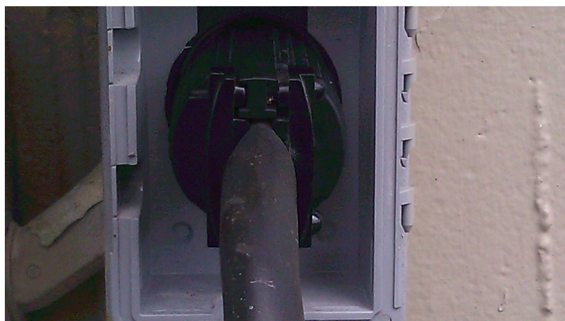
Figure 7. Emergency Power Input Connector.
