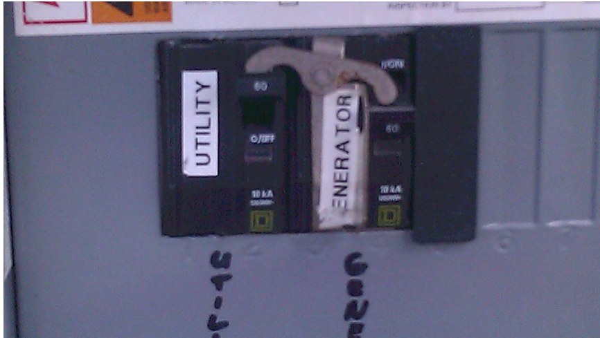
Figure 9. Circuit Breakers shown on Utility Power.
