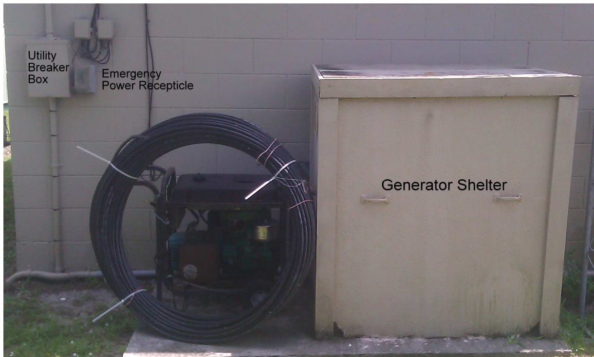
Figure 1. Utility Circuit Breaker Box, Emergency Power Receptacle Box, and Generator Shelter.
